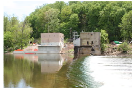
A water intake station on the Perkiomen Creek.
