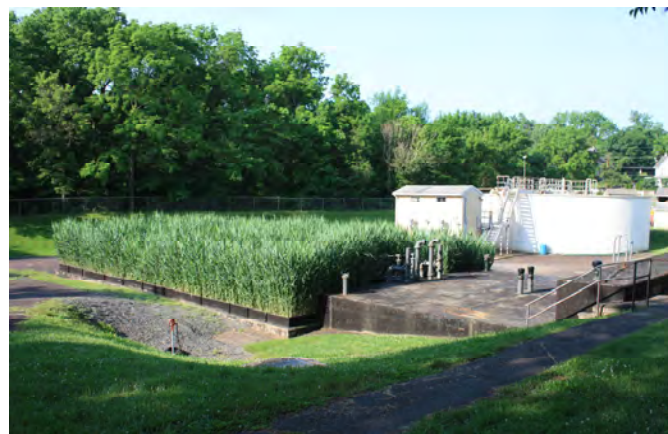
Schwenksville sewage treatment facility.
