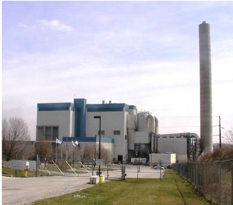
The municipal waste resource recovery facility contains several types of air pollution control systems to minimize air emissions.
