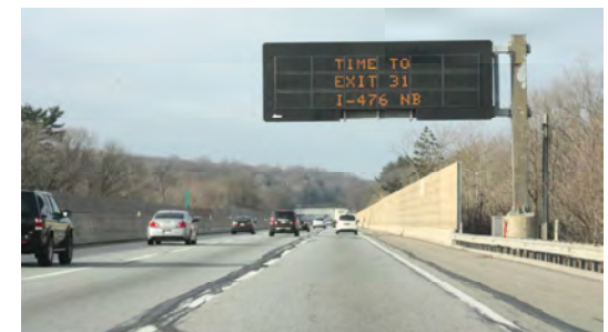
Variable message sign on WB Pennsylvania Turnpike (I-276) in Whitmarsh Township.
