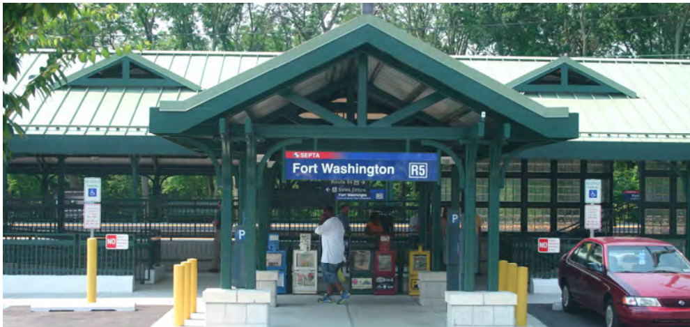
The newly rebuilt Ft Washington station along the Lansdale/Doylestown Line in Whitmarsh Township.
