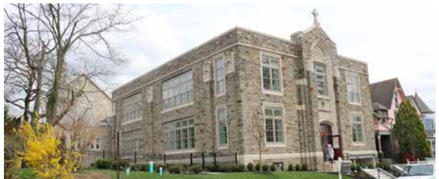
The former St. Margaret School in Narberth has been converted to condos.
