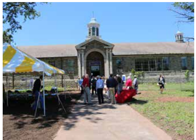
Groundbreaking for the adaptive reuse of the Perkiomen Valley Middle School, Trappe.
