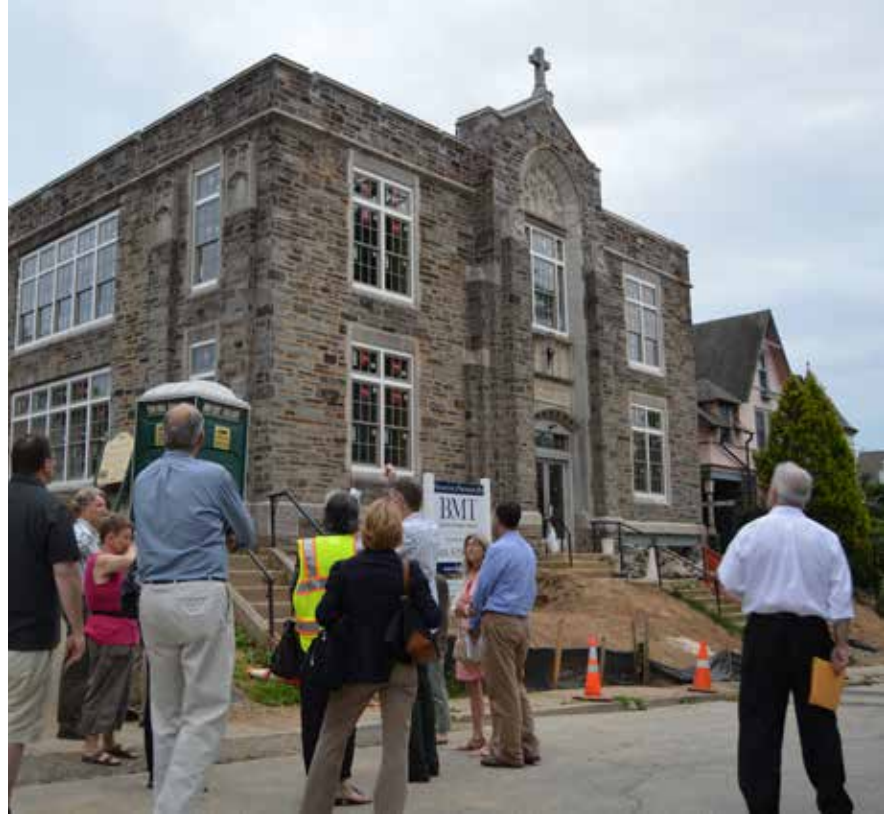
St. Margaret School during its conversion, Narberth.
