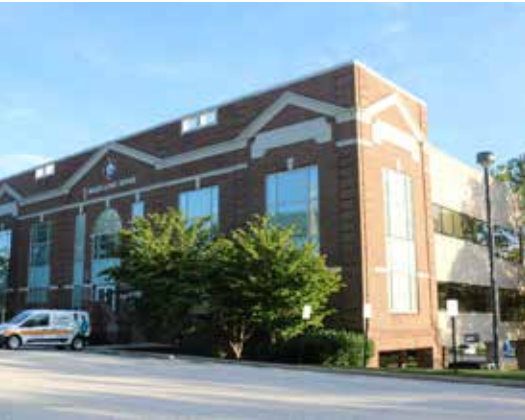
An addition with parking garage was added to the former Upper Merion High School.
