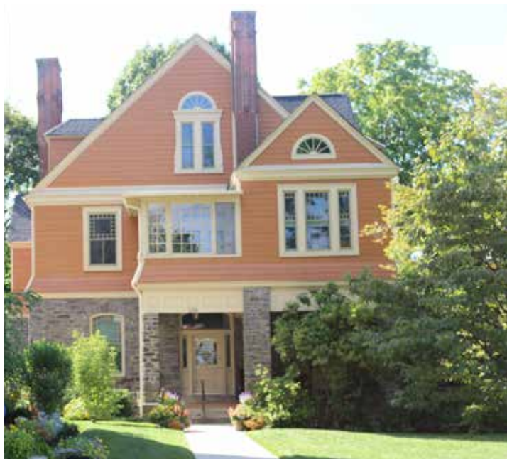
Previously the parsonage, Barrie House required extensive renovations.
