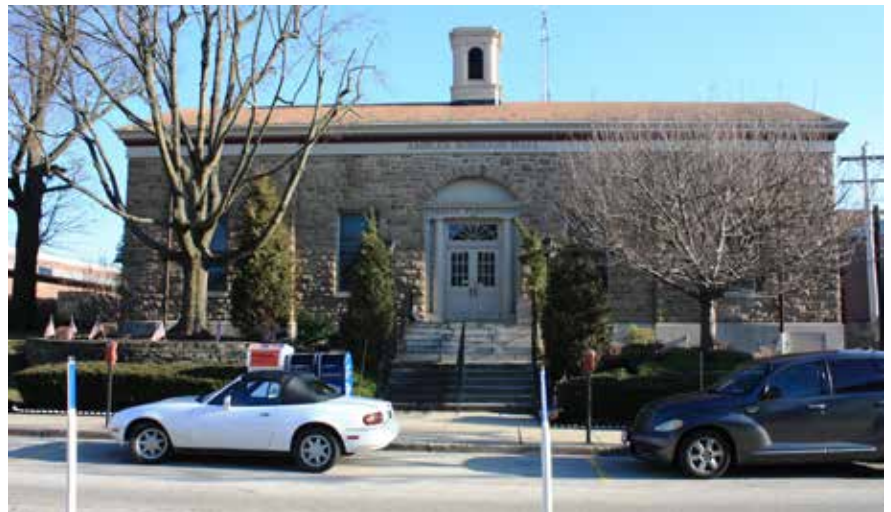
The former Ambler Post Office became the Ambler Borough Hall, and will be reused again as office space.
