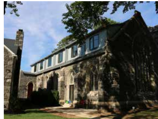
An accessible entrance (above) and second story dormers (below) were added to the former First Baptist Church, Lower Merion.
