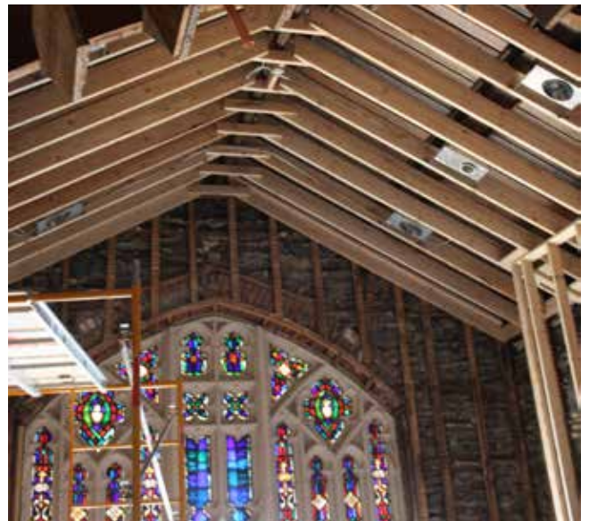
The striking stained-glass windows were restored by local craftsmen.
