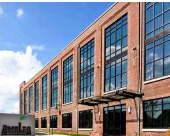
Ambler Boiler House, Ambler
