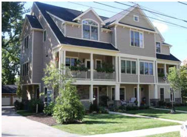
Newly constructed Vauclain Manor was designed to fit into the neighborhood.
