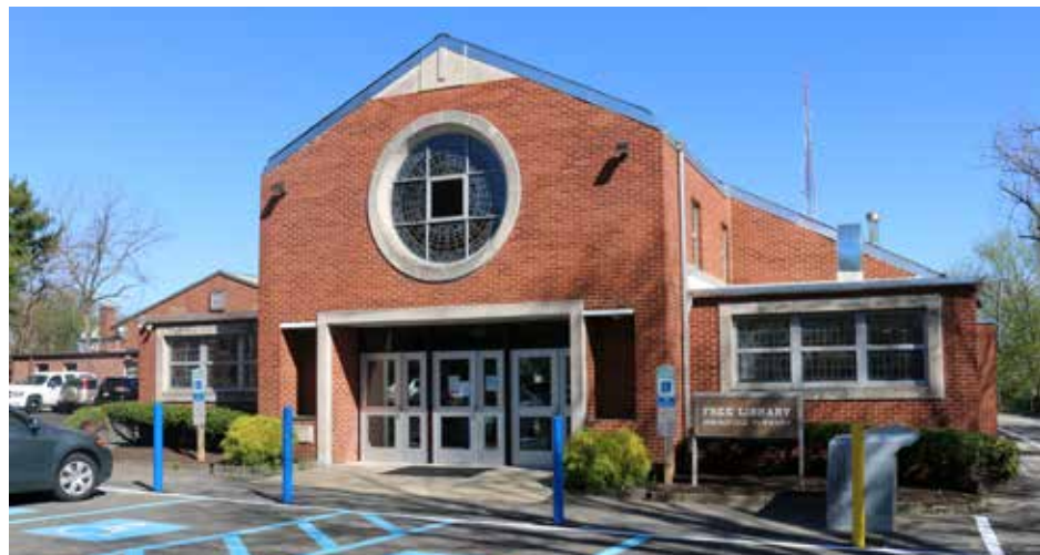
A handicap entrance was added and religious imagery was removed from the building.
