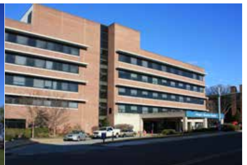
Abington Memorial Hospital, Abington.
