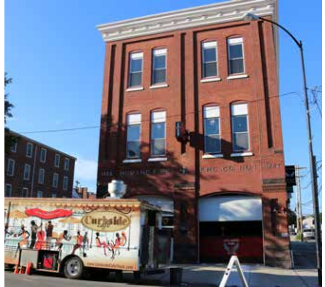
The adaptive reuse of the firehouse maintained an important building on East Main Street.
