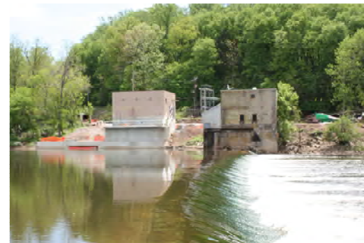
A sewage pump station on the Mill Grove side of the Perkiomen Creek.
