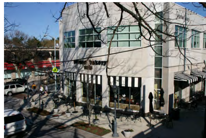
Mixed use building next to the Ardmore train station.
