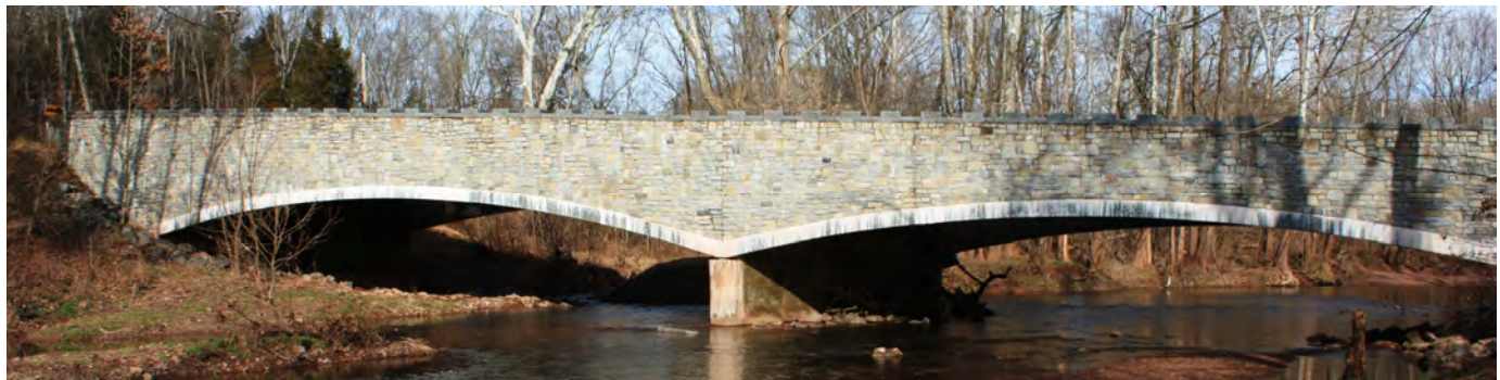
This new bridge along Kratz Road was designed in a context-sensitive way to be a good fit for its scenic surroundings.
