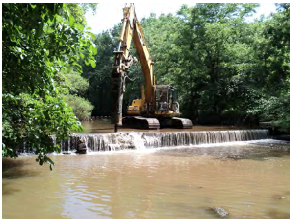
An old dam in the Wissahickon Creek is removed to improve water quality and fish habitat.
