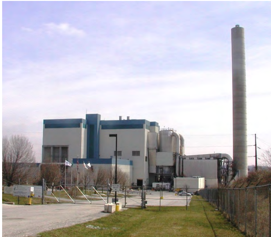
The municipal waste resource recovery facility contains several types of air pollution control systems to minimize air emissions.
