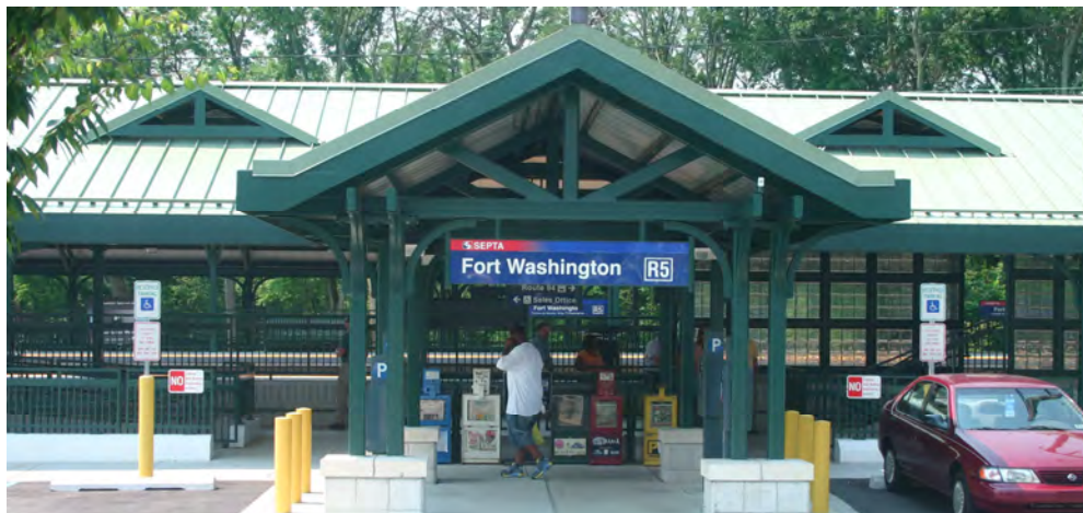
The newly rebuilt Ft Washington station along the Lansdale/Doylestown Line in Whitmarsh Township.
