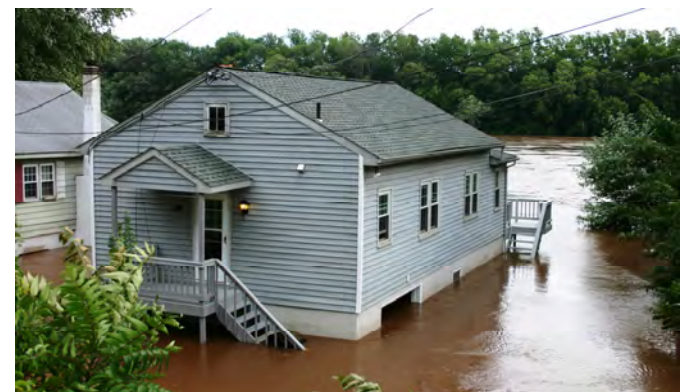
Flooding in the Port Indian community in West Norriton Township is a common occurrence.
