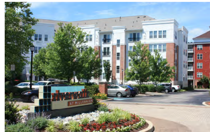
Dense residential development, such as the Riverwalk at Millennium apartments in Conshohocken, can help create a healthy balance between jobs and housing.
