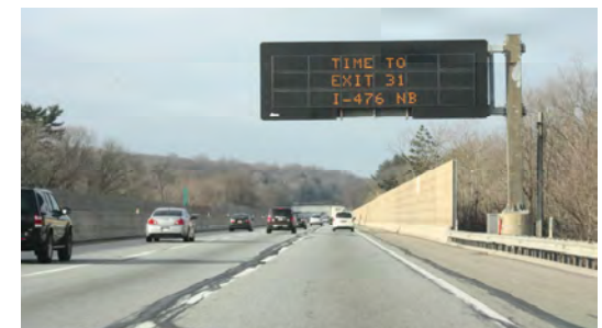
Variable message sign on WB Pennsylvania Turnpike (I-276) in Whitemarsh Township.
