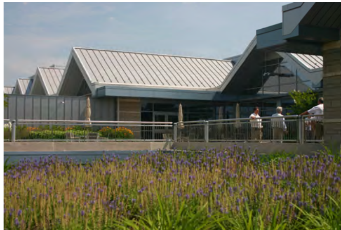
Environmentally-friendly office and research facility.
