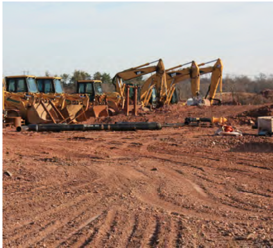
The grading of soil to prepare a site for development can be costly.
