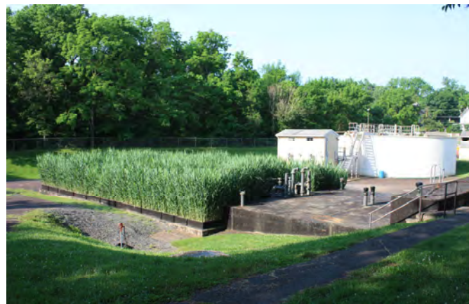
Schwenksville sewage treatment facility.
